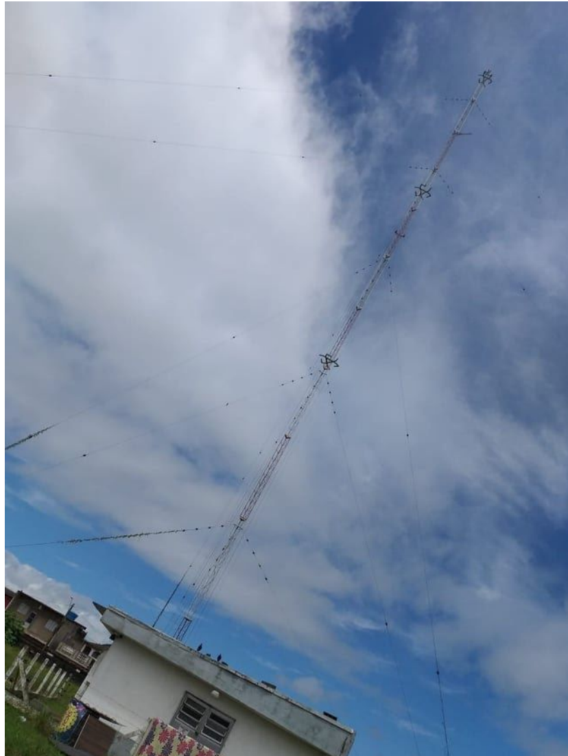
Photo: Antenna, folded monopole over 60 meters high.
